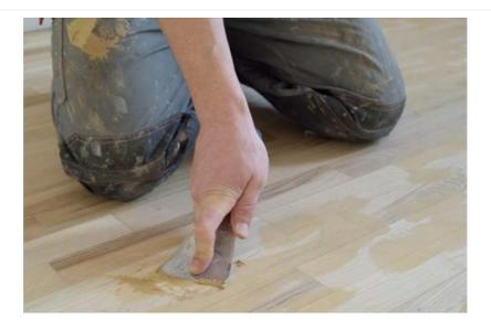
Finally, close the holes. Use a wood patch, putty, or other appropriate material to close or repair the holes made in the wood by your treatment.
