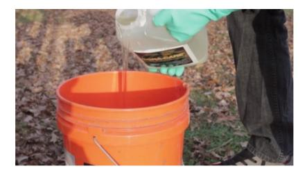
If you are treating wood that is currently infested, mix 1-part Bora-Care with 1-part water. Bora-Care should always be mixed in a 5-gallon bucket rather than directly in a hand pump sprayer because it will clog the sprayer if not pre-mixed with water. We highly recommend using hot water to mix with Bora-Care as the product is very thick and viscous and can be hard to mix.
