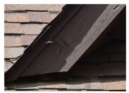
Carpenter bee damage is usually very conspicuous. Carpenter bees drill holes into wooden elements of structures, fences, lawn furniture, play structures and garden fixtures. Numerous carpenter bee holes can be very unsightly and costly to repair. Learning to spot carpenter bee nests early can help you limit the damage the bees cause.
