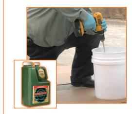
Use a drill and impeller to mix Bora-Care with Mold-Care
