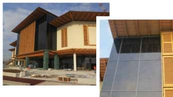
Even before construction was completed pigeons started to roost in sheltered parts of the building. Pigeons roosting below the roof were creating an unsightly mess on the glass façades
