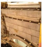
At the second floor, all nests were removed from below the curved lintel above the central window, from below the inverted V-shaped lintels on either side and from the architectural features to left and right. All these surfaces were treated with dishes of Optical Gel at 6 in centers to prevent nesting.
