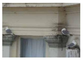
Optical Gel dishesapplied to the façade above the main entrance are invisible from below
