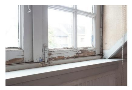
Wood Decay fungi are living organisms which feed on damp wood and cause the damage known as rot. Decay fungi send tiny threads called hyphae through wood, breaking down the wood fibers and making them weak and brittle. The term "dry rot" refers to the effects of such damage rather than the cause: dry wood will not rot. Excessive moisture is the primary cause of rot since wood decay fungi will transport water through wood to dry areas, weakening and possibly destroying wood.
