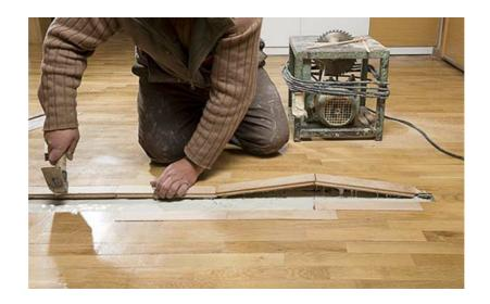
If you have wood that was previously infested with woodworms or wood-boring beetles, the structure of the wood may be compromised due to holes and tunnels from the woodworms. Replace the wood if possible. Replacing wood may also be a more economical option than treating the wood if only one or two pieces of wood were infested.
