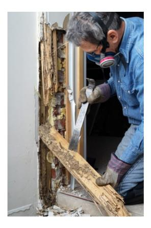
The simplest way to get rid of drywood termites is to remove and/or replace infested wood. If the infestation is localized to one or two pieces of easily accessible wood, you can simply remove and replace the infested wood to effectively get rid of drywood termites in your home. If the wood cannot be removed or replaced, see the methods below for treatment options.
