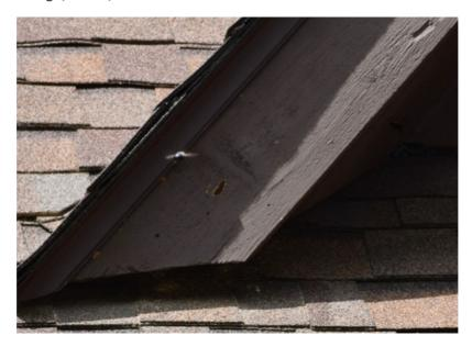
Carpenter bee damage is usually very conspicuous. Carpenter bees drill holes into wooden elements of structures, fences, lawn furniture, play structures and garden fixtures. Numerous carpenter bee holes can be very unsightly and costly to repair. Learning to spot carpenter bee nests early can help you limit the damage the bees cause.
