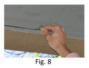
Adjust the nozzles after the tube is installed to get your desired spray angle.
